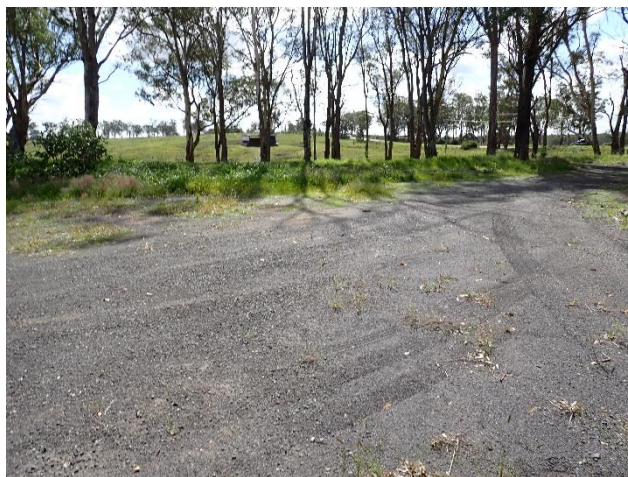
Figure 12 – Disturbed bitumen area in central portion of SU2. View north.
