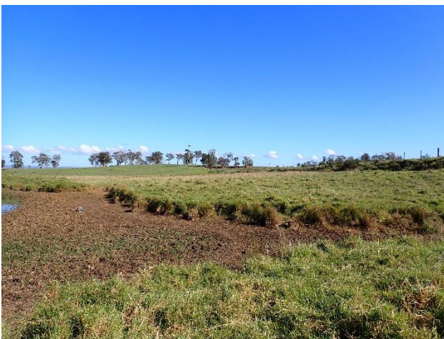
Figure 49 – Photo of high disturbance in dam embankment area in central portion of SU4.
