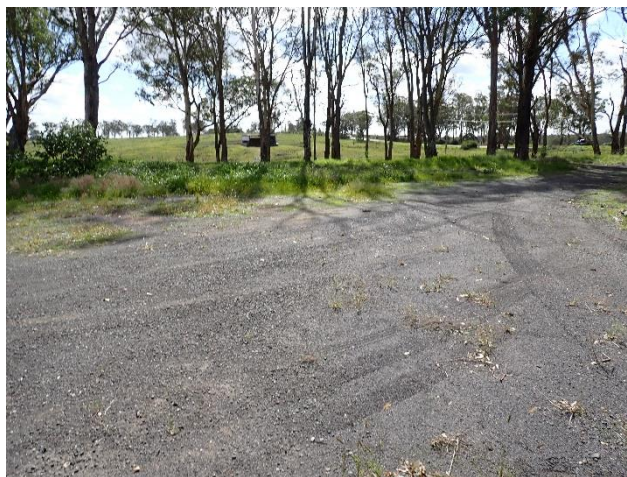
Figure 12 – Disturbed bitumen area in central portion of SU2. View north.
